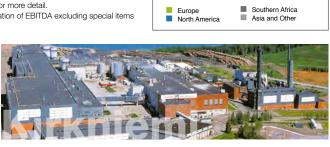
A new power plant, at Kirkniemi Mill, expected to be operational early 2016, will significantly improve cost competitiveness and profitability by reducing energy costs and securing energy supply. The plant can potentially use 100% solid biomass such as bark from the mill's debarking process.
