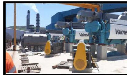
New Wash Presses in position
