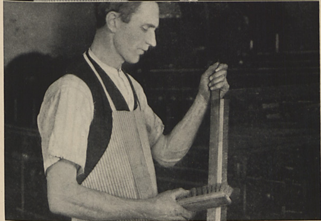
THESE pictures show cleaning of press brush. Press brush is scrubbed back and forth with hand brush. After this it is tamped with back of hand brush to remove all loose particles before putting back on press
