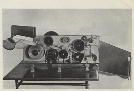
STANDARD POSTAL PERMIT PRINTER AND SEALER OPERATION No. 1 After laying the envelopes flap down, the operator adjusts the horizontal feed so that the bottom envelope feeds smoothly over the large roll at left of picture
