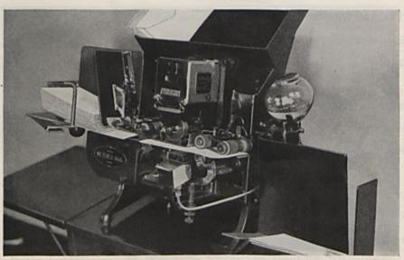
PITNEY-BOWES MODEL "B" Immediately after printing the indicia, the moistening and sealing of the flap begins. The smooth, easy operation of the Warren's Standard Booklet Envelope at this point is very pleasing to the operator
