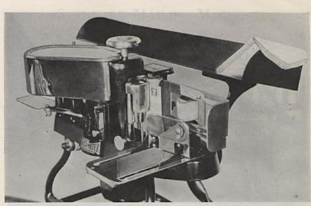
PITNEY-BOWES MODEL "AM" OPERATION No. 3 Another view of the MAIL-O-METER, to show the position of stamped envelope (almost the exact center of the illustration) coming smoothly through pressure rolls after sealing and stamping
