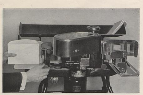
PITNEY-BOWES MODEL "AM" OPERATION No. 1 Setting the guide for envelopes in the MAIL-O-METER Stamp Affixing Machine. For this vertical feed machine the flaps are opened and well extended for easy riding over the feeding guide which the operator is adjusting
