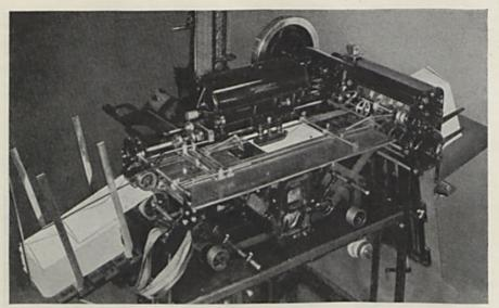
ADDRESSOGRAPH MODEL "A-4" OPERATION No. 4 An all-operation view showing envelopes leaving the machine and being stacked at the left of the illustration. Note also that another envelope is approaching printing position
