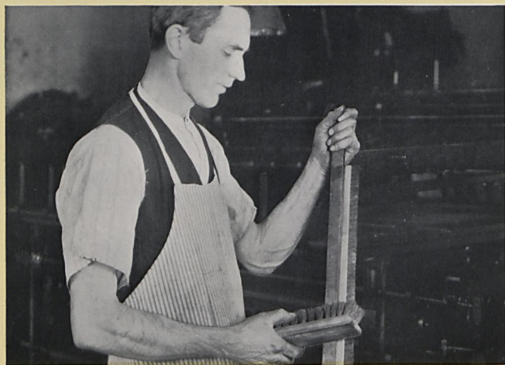
THESE pictures show cleaning of press brush. Press brush is scrubbed back and forth with hand brush. After this it is tamped with back of hand brush to remove all loose particles before putting back on press
